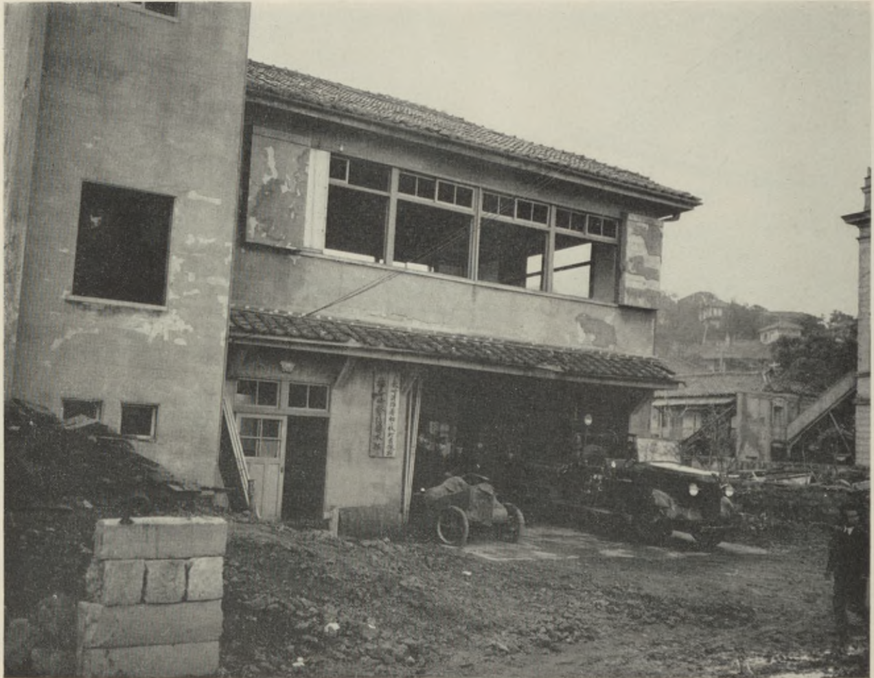
Photo 11. Matsugae Substation. Partially damaged by atomic bomb of 9 August 1945.
